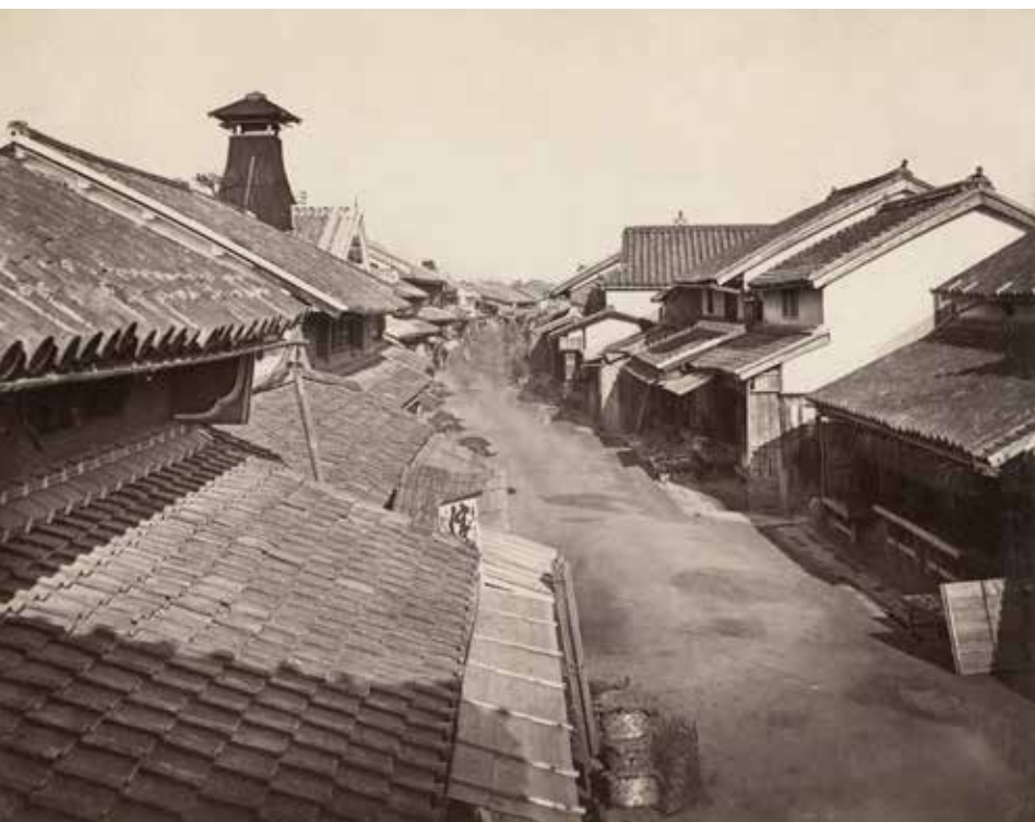
LEFT. 52. Nakamachi on the Saigoku Kaidō Road in Kobe. The building with the fire lookout tower is the Kobe Town Hall, formerly the Kobe Village Assembly. Near this building was an entrance way to Zenshōji.
