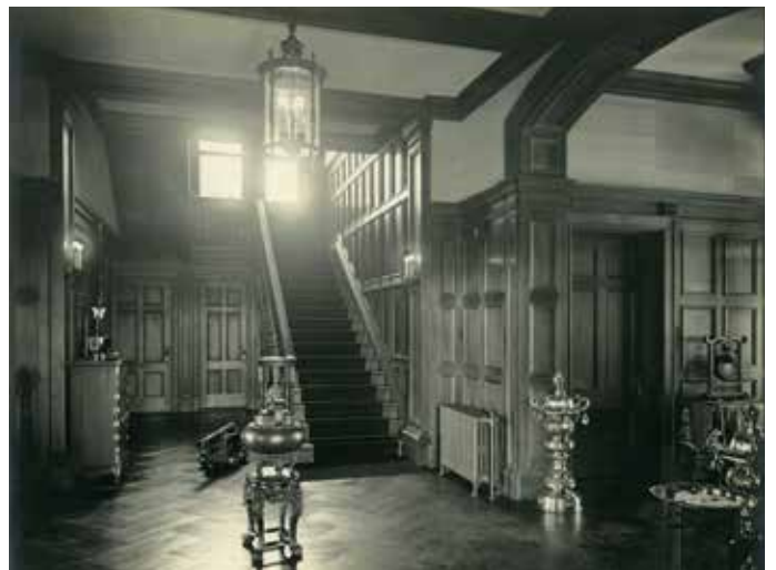
39. Entrance hall with stairs to the second floor.
